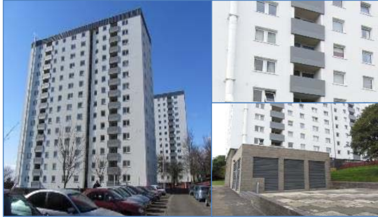
Dallfield Multi-storey development
