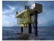
2008 PS100 Installation in the River Humber
