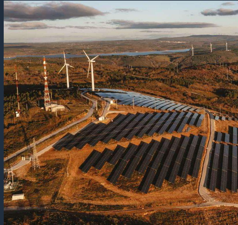
Hybrid power plant. Source: EDPR
